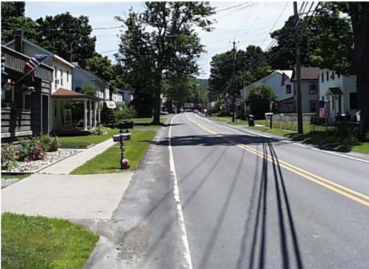
Sidewalk on left ends at end of property line. Sidewalks should be continuous to encourage their use.
